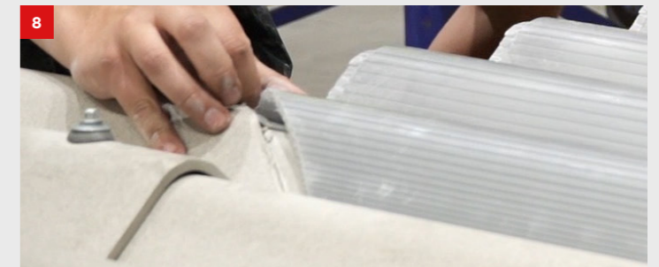
Make sure to mitre the appropriate corners depending on the direction which you are laying the sheeting. The mitre measurements will be the same as if it was a fibre cement sheet.
