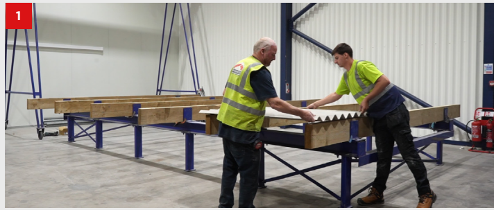
Lay the first run using our Big 6 fibre cement profiled sheeting.
