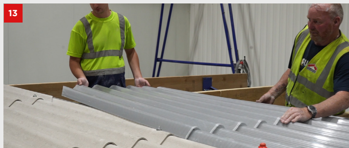
Continue to install the Heatguard 50 sheets accordingly.
