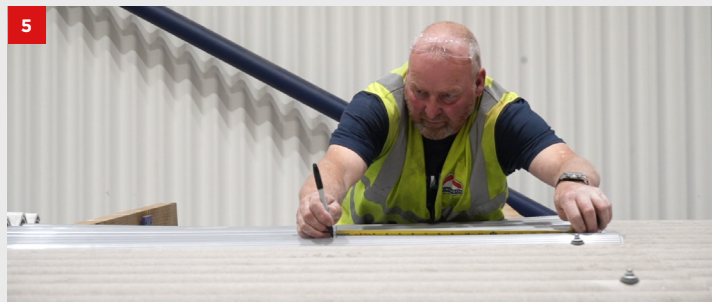
The secondary fixings should be positioned at 450mm between each fixing on the side lap corrugation.
