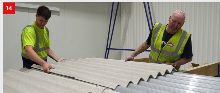
The entire ridge course should be laid using fibre cement sheets to ensure that the Heatguard 50 sheets are truly square to the fibre cement profile. These sheets should be fixed in accordance to the design guide.
